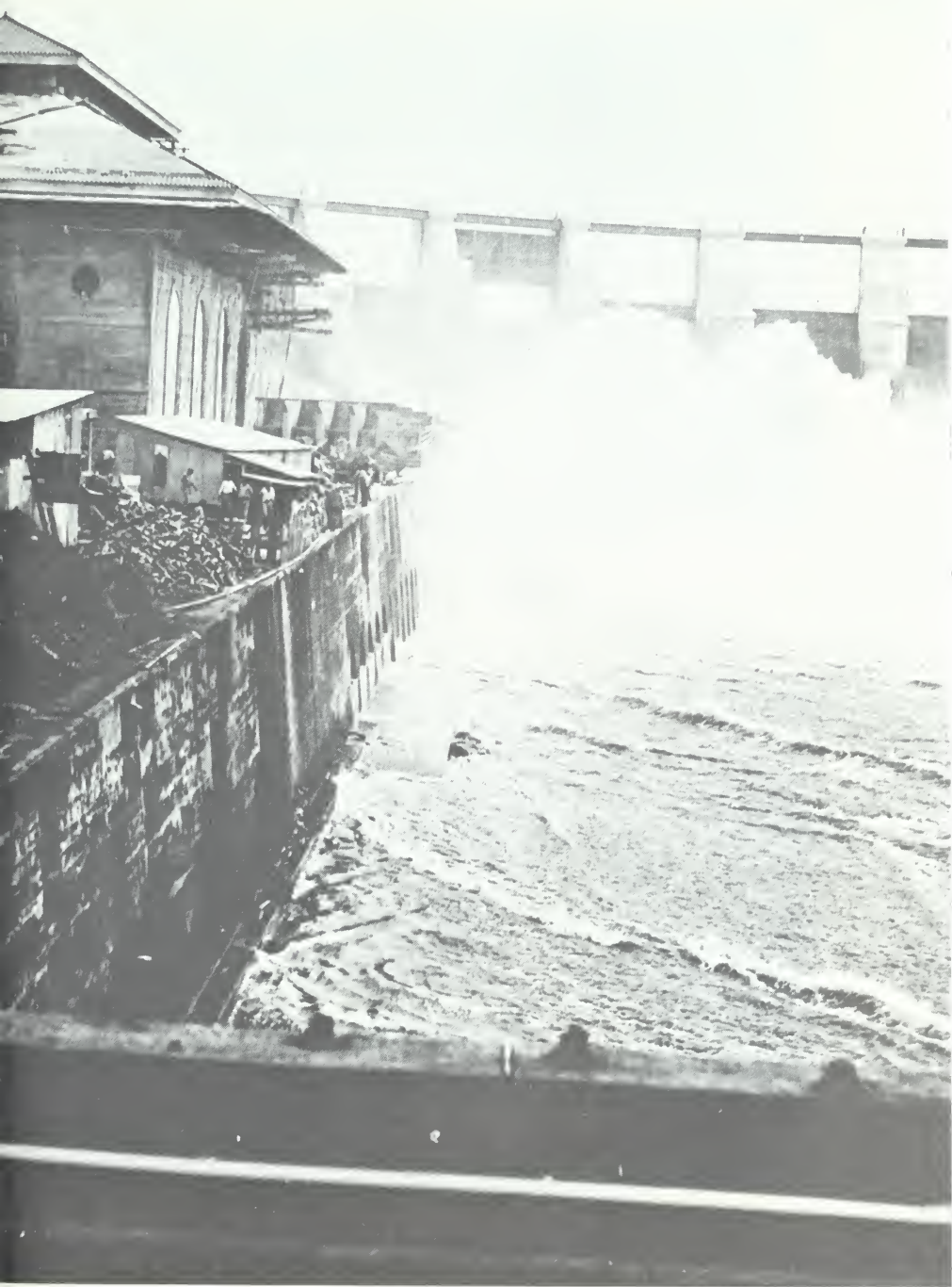
Left and above: Filling Gatun locks for the first time. The building in the upper left corner is the control house from which all the machines on the locks were controlled
